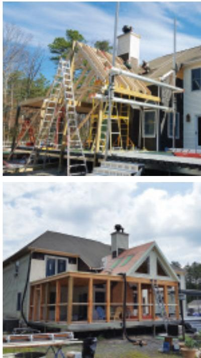
**Figure 3.** Support columns for the sunroom bear either on the house foundation or directly on piers (top). The structure was timber-framed with a combination of pressure-treated sawn and engineered lumber (above).
