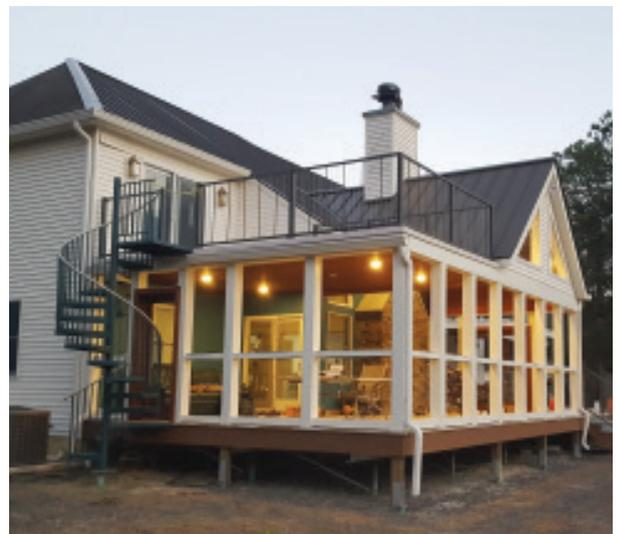
**Figure 6.** For low maintenance, the porch trim and the balcony trim were wrapped with PVC-coated coil stock, while Trex fascia trim was used to finish the edge of the deck and the stair stringers (top). The aluminum vertical cable railings are Digger Specialties' Westbury VertiCable (above).
