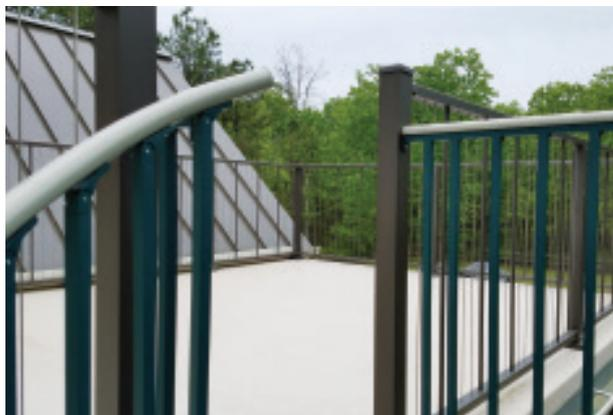
**Figure 5.** The lower deck is finished with travertine stone that was glued around the perimeter to the steel framing with two-part epoxy. In the field, the pavers were dry-laid, and the joints filled with polymeric sand (top). A subcontractor installed waterproof fiberglass walking surfaces on the two upper decks (above).
