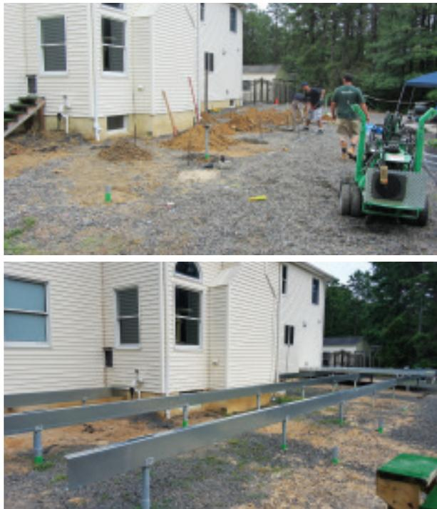
**Figure 1.** Instead of massive concrete footings, helical piers—each capable of supporting 5,000 to 8,000 pounds—were installed to support the freestanding deck (top). The 6 $\frac{1}{4}$ -inch Paverdeck panels are screwed to galvanized 10-inch LGS steel beams bolted to the brackets on top of the piers (above).
