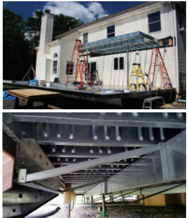
**Figure 2.** The LGS joists on the upper deck hang from galvanized rim track with preformed, prepunched tabs at standard spacings (top). Diagonal bracing was installed on the lower deck to solve a pesky vibration problem in the steel deck framing (above).
